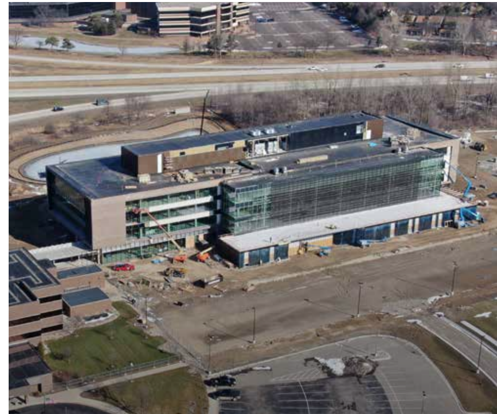
progress on the south campus building
